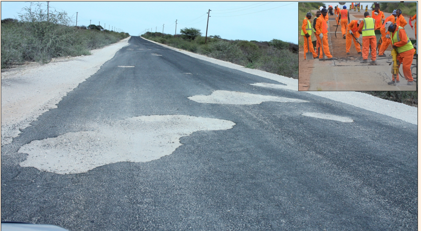
Routine maintenance especially in the form of pothole plugging on roads often pose a challenge but plans are in place to deal with the challenges adequately to make most pothole-infested roads like the one below trafficable
