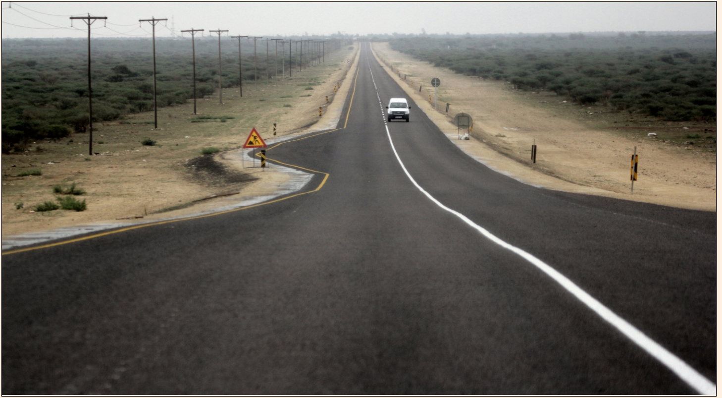
This is a completed road, one of the Capex projects Kagisano Molopo District, Dr Ruth Segomotsi Mompati District. It is from Morokweng to Vostershoop.
